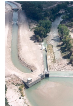
Figure 1. Fully automated Swasey Diversion Structure with flow and water level monitoring
