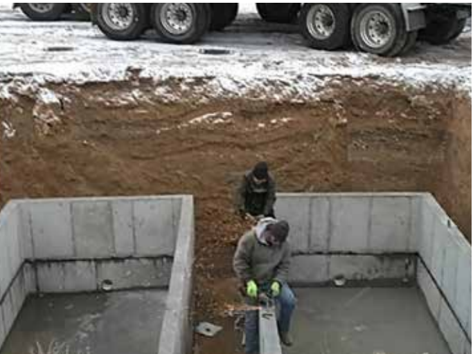
Above: Construction on the 10,000 gallon water tanks in Shambip District.v
