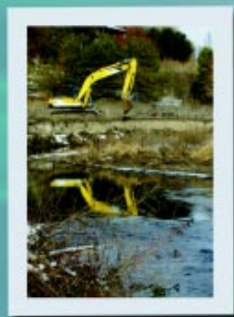
Construction was under way in December 2000.
