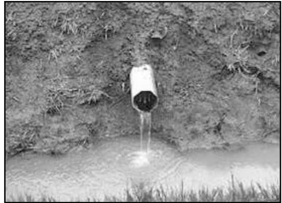
A field drain empties into a drainage canal.
